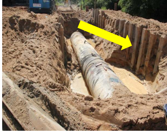
Gambar 4.2 Temporary Interlocking Sheet Pile
